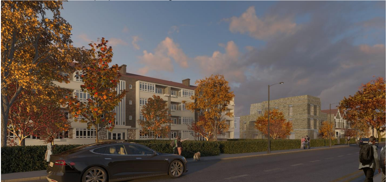
Fig 4- View along Park Road
